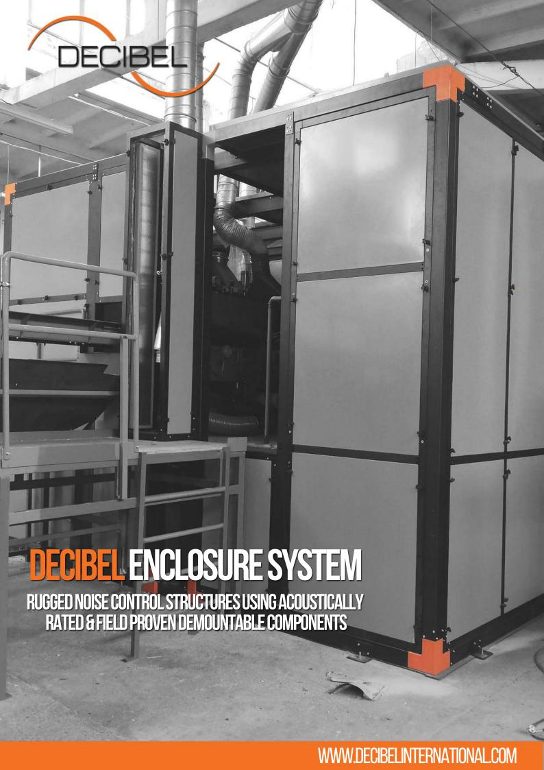
**DECIBEL** Dbox<sup>®</sup> enclosures protect workers from noise generated during manufacturing. In industrial settings, noise from equipment frequently exceeds limits for hearing safety, while also impeding communication. Without noise control remediation, local noise ordinances at plant property lines may be exceeded.
